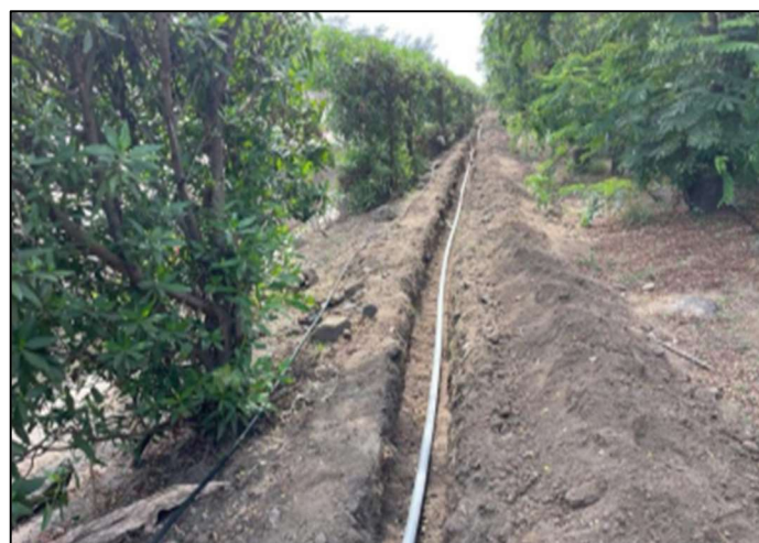
Photo of Drip Irrigation system for green belt development
