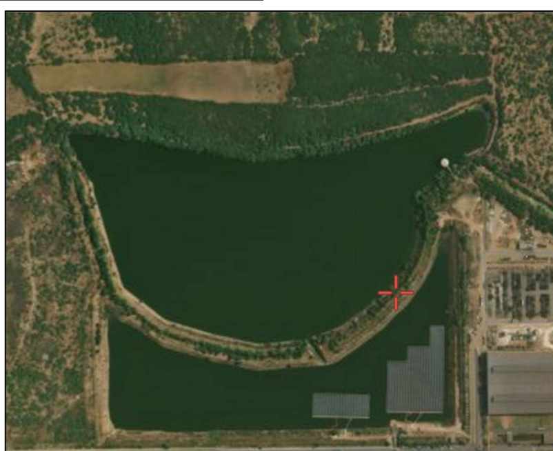
Satellite view of Rain Water Harvesting Pond
