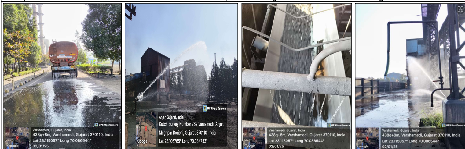
Geo-tagged photographs of water sprinkler system at coal storage area, other open storage area and material conveying belts and also deployed water tanker
