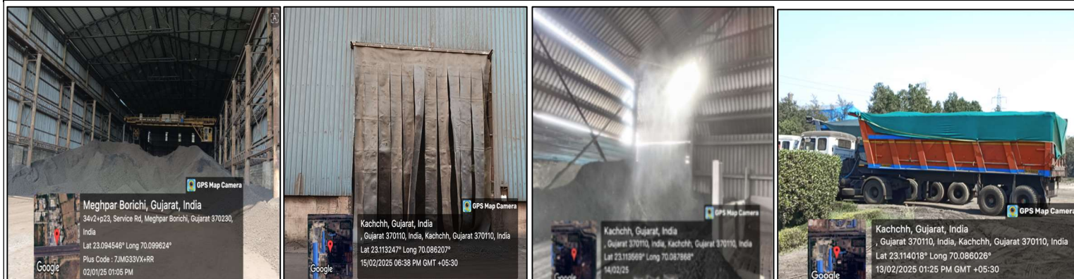
Fully Covered shed facility for the Coal handling & Storage, Fogg spray system and covered trucks
