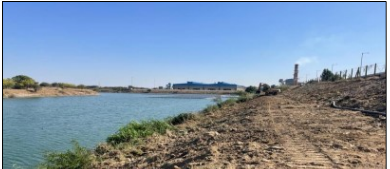
Photographs of rain water harvesting pond
