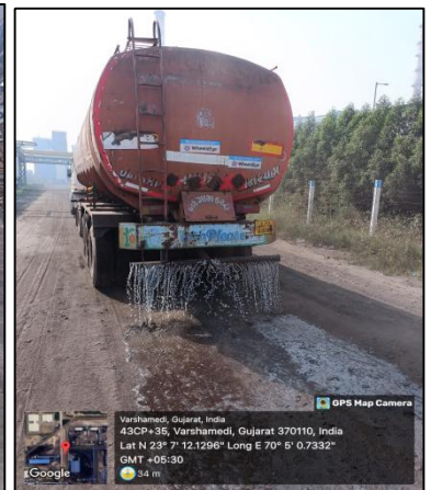
Photos of water spraying for the dust suppression
