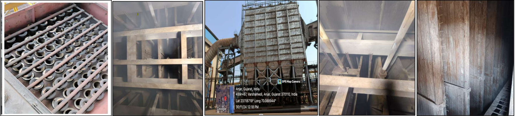
Photographs of the Maintenance of ESP fields & Bags replacement in Air Pollution Control Devices (APCD)
