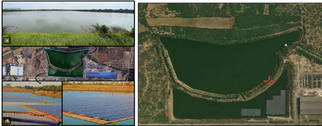
Satellite view of Rain Harvesting Pond
