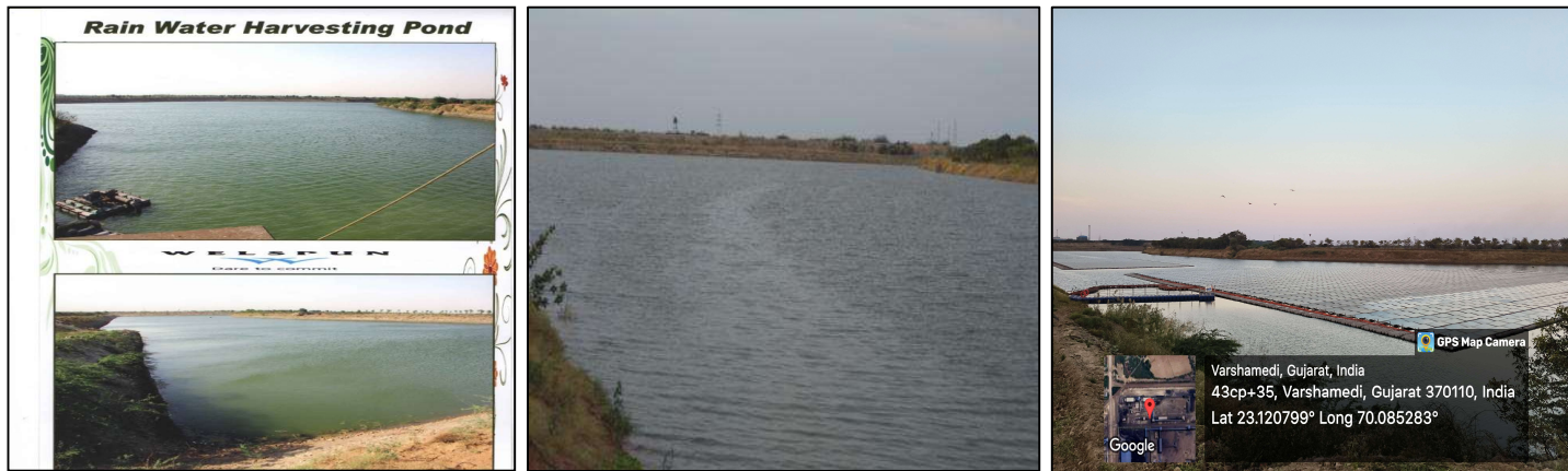
Photographs of Rain Harvesting Pond
